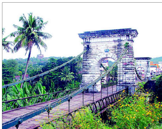
Punalur Suspension Bridge
