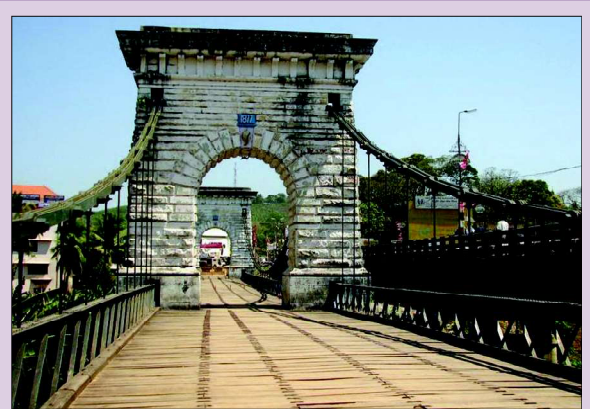
Punalur Suspension Bridge
