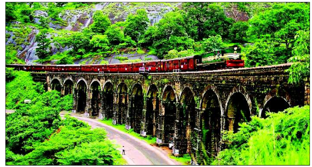
Meter gauge rail way line (Pathimunnu Kannara Palam)
